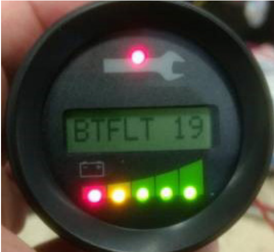
Battery Fault Display
