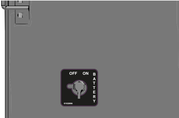
Figure 3.1.1: Battery Disconnect Switch
