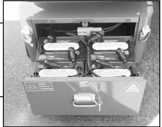
Figure 10: Access to Batteries
